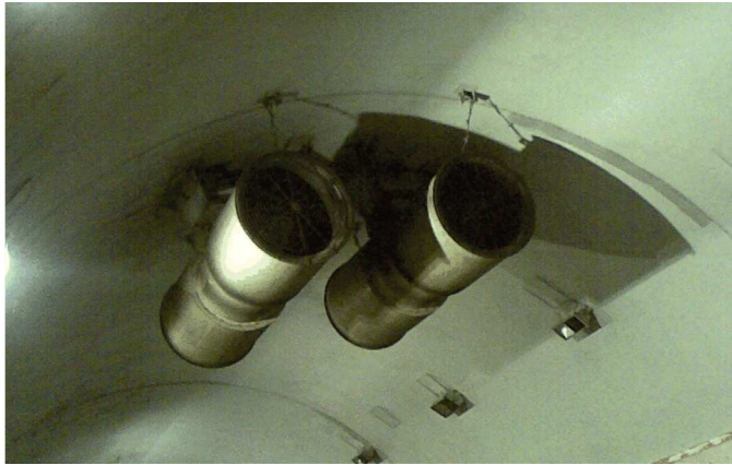
Fig. 8. Installed SDS112T-4P-22 jet fans in tunnel.
