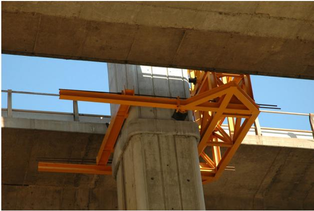
Figure 21. Fastening of the auxiliary metal structure to the concrete pier.
