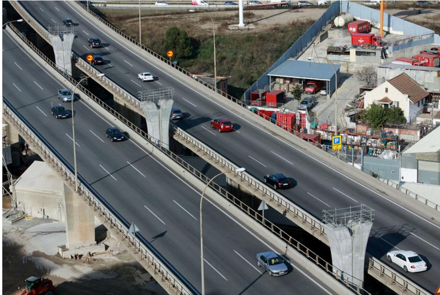
Figure 17. Viaduct piers, installed before building the deck.
