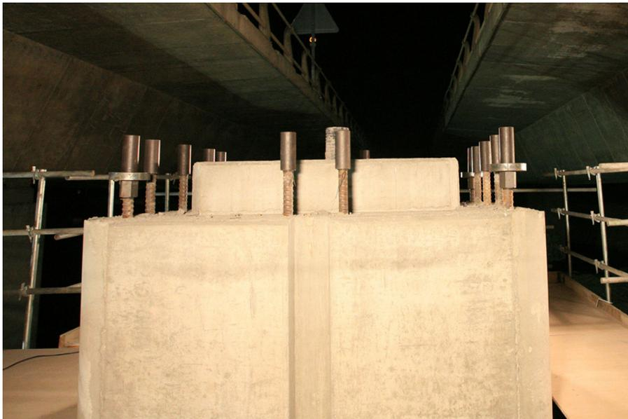
Figure 15. Upper part of the fraction of pier built *in situ*. You can see the 50 mm diameter vertically protruding bars placed prior to the operation for mounting the upper prefabricated piece. Compression nuts on the corner bars and bearing pads are placed below the couplers. Only stress bar couplers were placed on the remaining bars.
