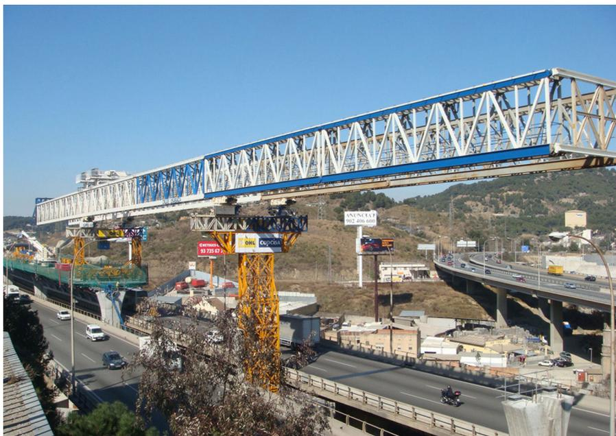
Figure 18. Launching girder measuring 120 m long, with cantilevered front end.
