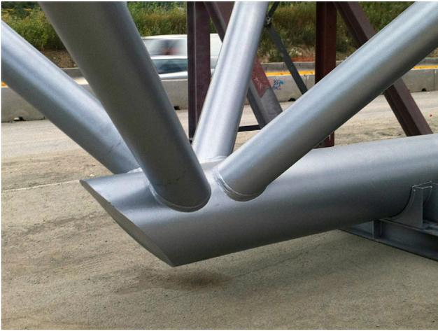
Figure 9. Joint on one of the ends of the lower chord of the latticework.
