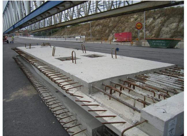
Figure 12. Prefabricated deck slabs.
