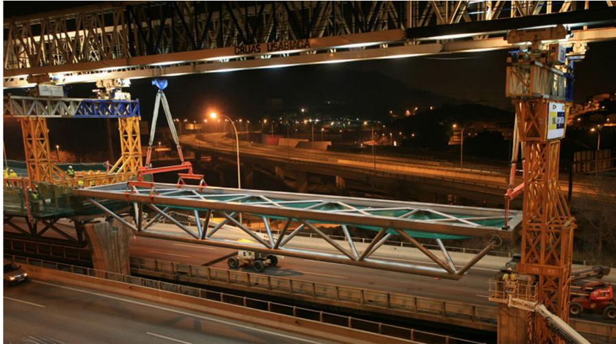
Figure 25. Placing a lattice girder into its final position using the launching gantry.
