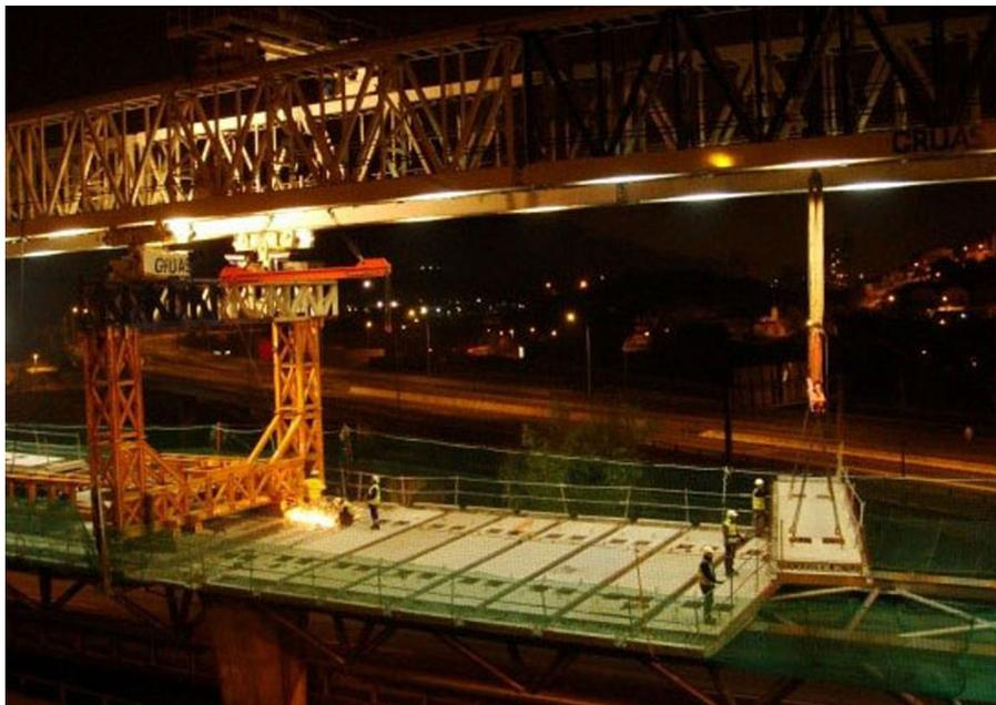
Figure 26. Mounting the prefabricated slabs with the launching gantry.
