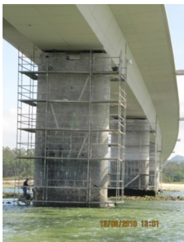
Cathodic protection wiring installation of a pile
