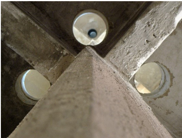
Figure 5. Space for new columns through existing slabs.
