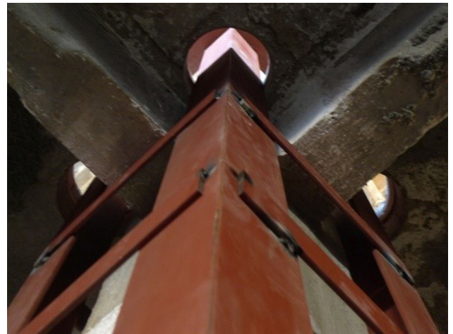
Figure 6. Already executed columns passing through the slabs.
