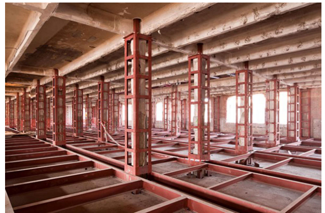
Figure 7. New steel structure in warehouse 8.
