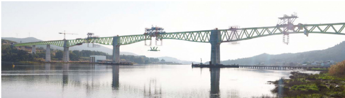
Figure 44. Hoisting the joining segment for span 7.
