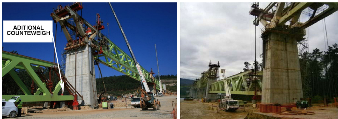
Figure 28. Hoisting sequence for spans 11 (left) and 10 (right).
