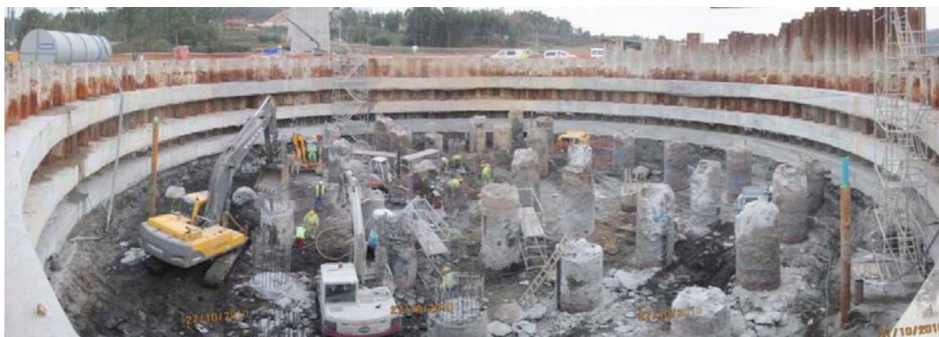
Figure 9. Cutting down P5 foundation pile heads.
