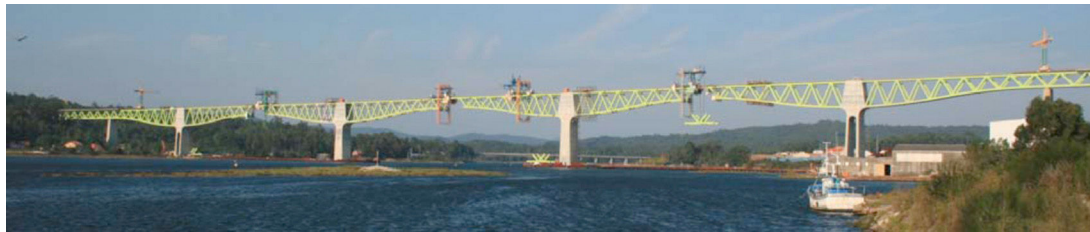
Figure 42. Hoisting the joining segment for span 6.
