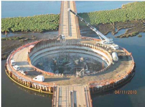
Figure 8. Inner excavation in P5 enclosure.
