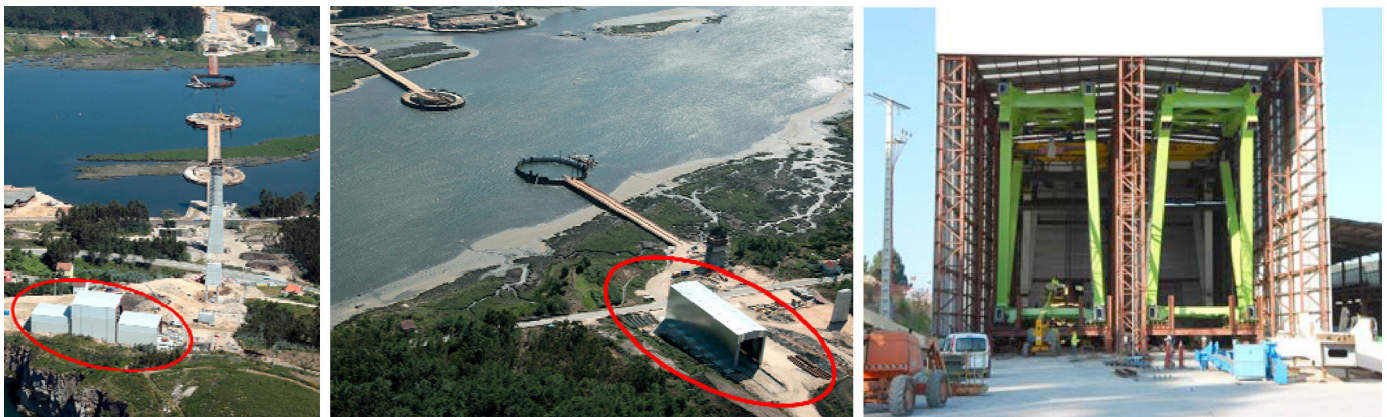
Figure 14. On-site segment assembly bays.
