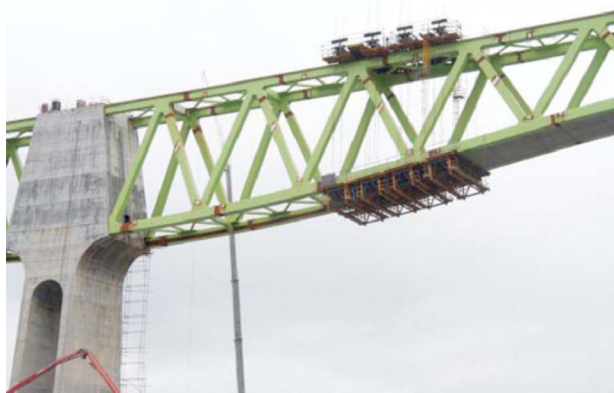
Figure 45. Travelling formwork for casting bottom slab concrete.
