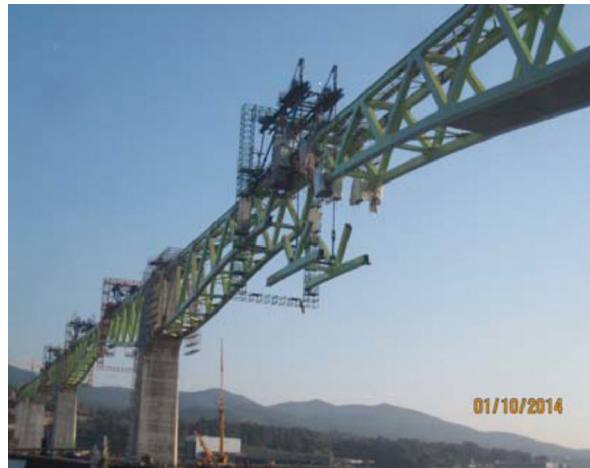
Figure 43. Hoisting the joining segment for span 8.
