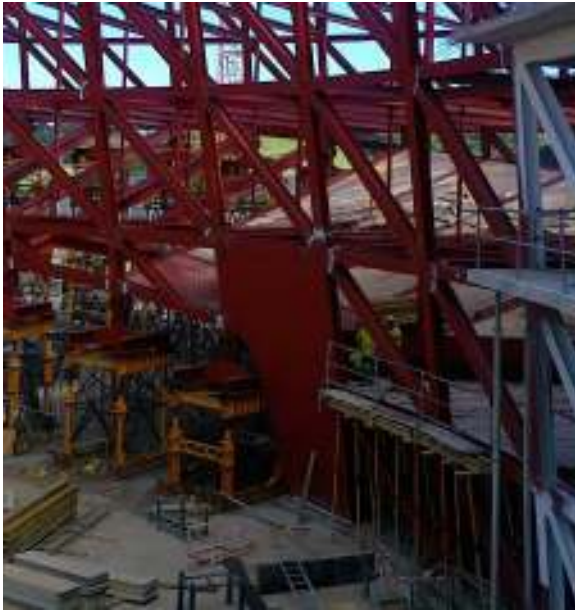
Figure 18. Reinforcing infill on the inner truss.
