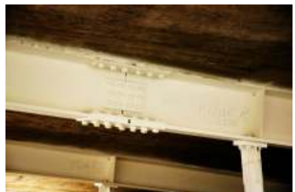
Figure 22. Bolted beam and beam-column joints.
