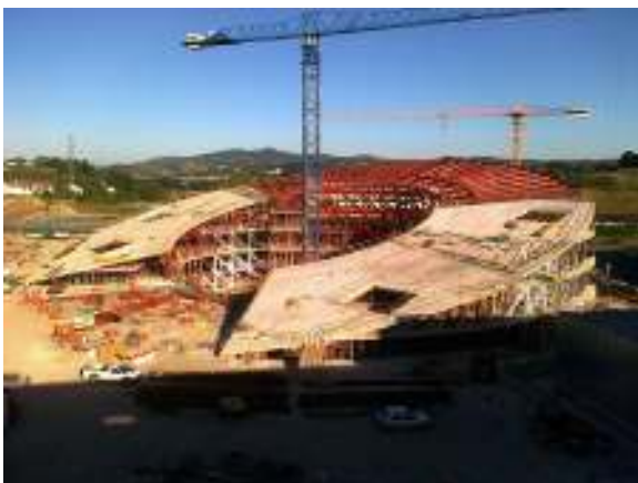
Figure 11. Construction of structural roof slab.
