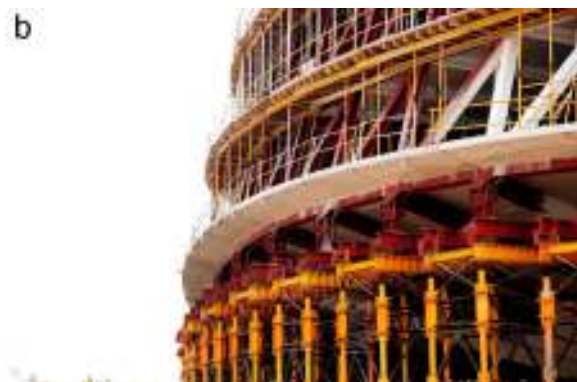
Figure 25. Alignment of the outer truss resting on provisional shoring towers.
