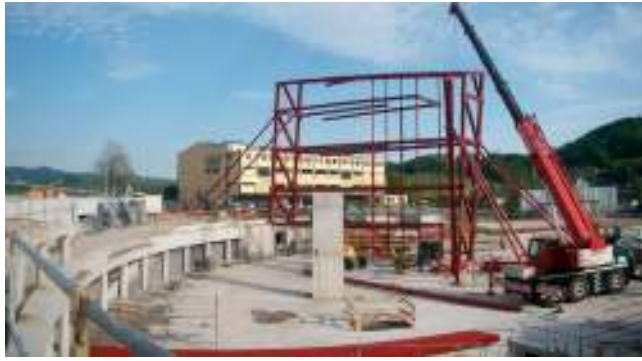
Figure 23. First structural sector, including two opposite truss panels, beams, and intermediate columns, as it was hoisted into position.
