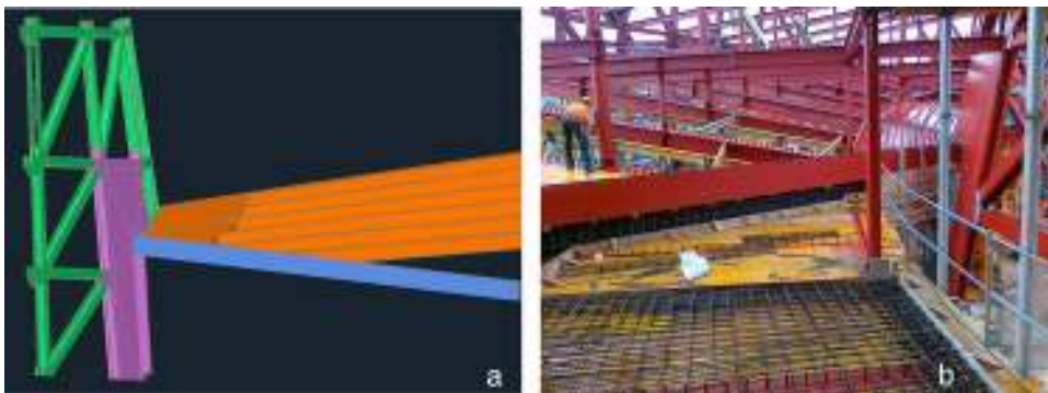
Figure 19. Reinforcing sheet metal on the bottom slab: 3D model simulation (left) and construction photograph (right).
