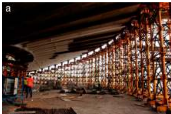
Figure 25. Alignment of the outer truss resting on provisional shoring towers.
