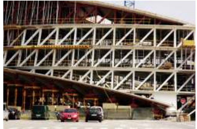
Figure 8. Side view of the outer truss during construction of the structural roof slab: note that the diagonals remain straight at the junction with bottom and roof slabs.
