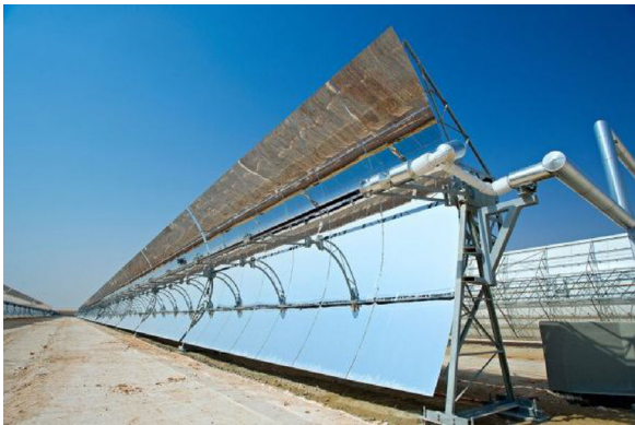
Fig. 8. Concentrated solar system for steam production (parabolic trough) (by Masdar Official (Shams 1 Parabolic Trough in Abu Dhabi) [CC BY-SA 2.0 ( https://creativecommons.org/licenses/by-sa/2.0 )], via Wikimedia Commons).
