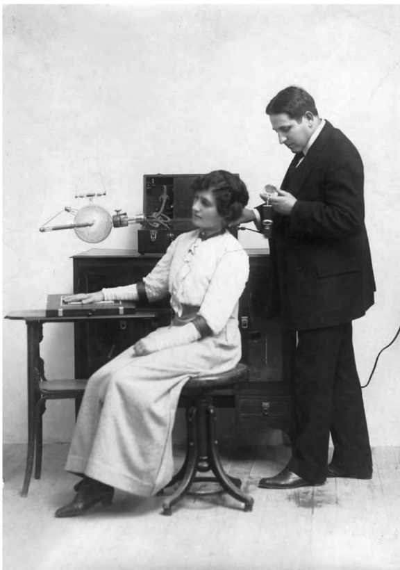
Figure 7 Scene with the Sánchez machine operated by Mónico himself, taking an X-ray of a woman's hand. Note the size of the briefcase and the Crookes tube mounted on a folding support. Photograph kindly provided by the family of Mónico Sánchez Moreno.
