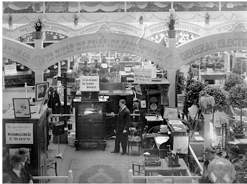
Figure 4 Photograph of the stand where the machine was exhibited under the make Collins-Sánchez, at the 3rd Electrical Show held at New York's Madison Square Garden in September 1909. Photograph kindly provided by the family of Mónico Sánchez Moreno.
