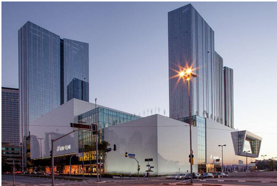
Fig. 2 – Shopping JK Iguatemi, São Paulo, SP – Brazil. Building characterized by the use of a ventilated facade with porcelain tiles.
