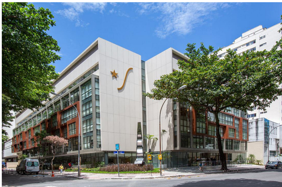
Fig. 5 – Copa Star Hospital, Rio de Janeiro, RJ – Brazil. Ventilated facade composed of porcelain tiles.
