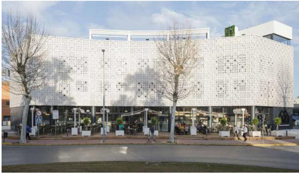
Fig. 7 – Alquería Market in Dos Hermanas – Seville. Ventilated facade made of polymer concrete. Source: Ulma [69].
