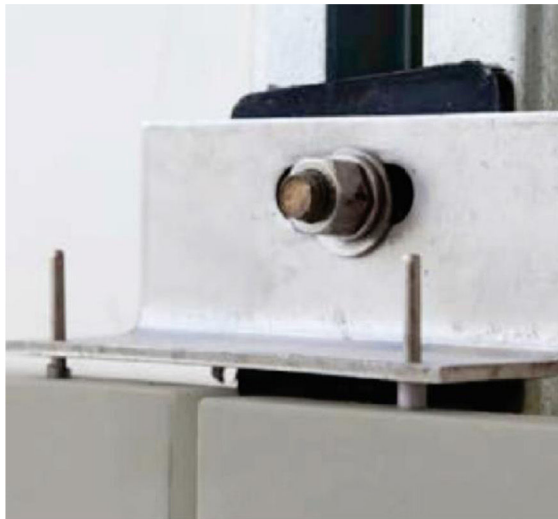
Fig. 8 – Detail of the fixing system with metal inserts – ELIANETEC. Source: Eliane [16].
