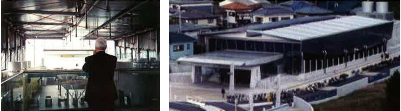
Figura 4. Nihon university subway station (Referencia [1])
