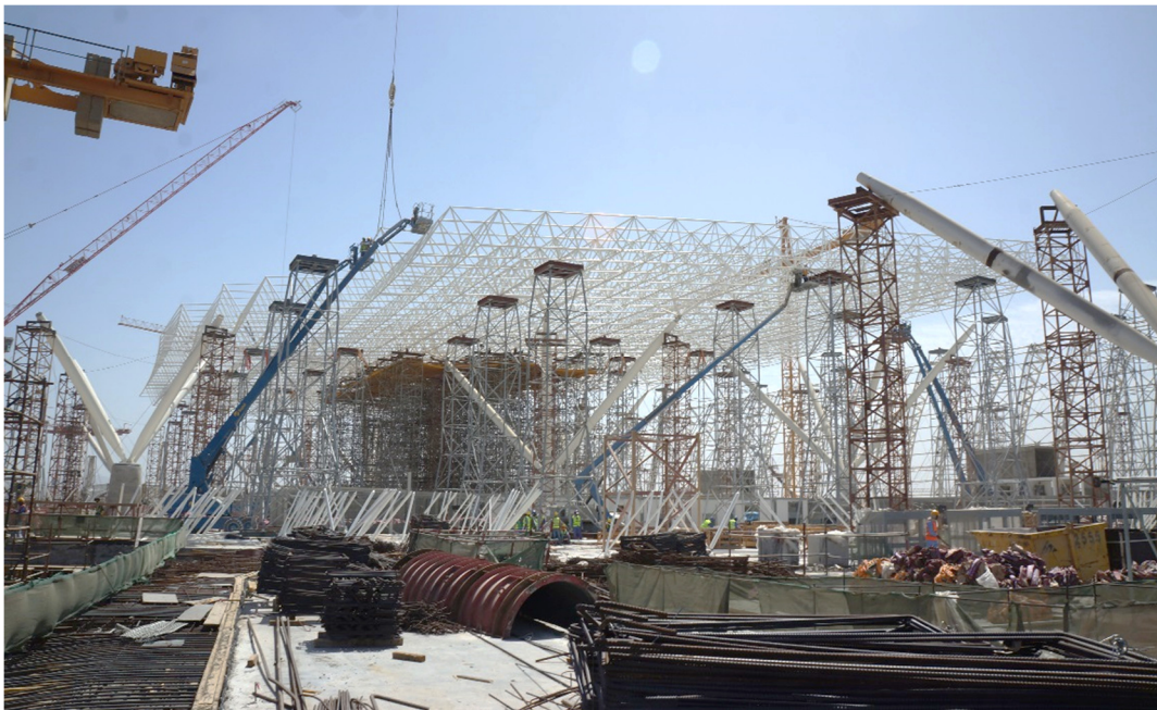
Figure 9. Processor, construction of the space frame.
