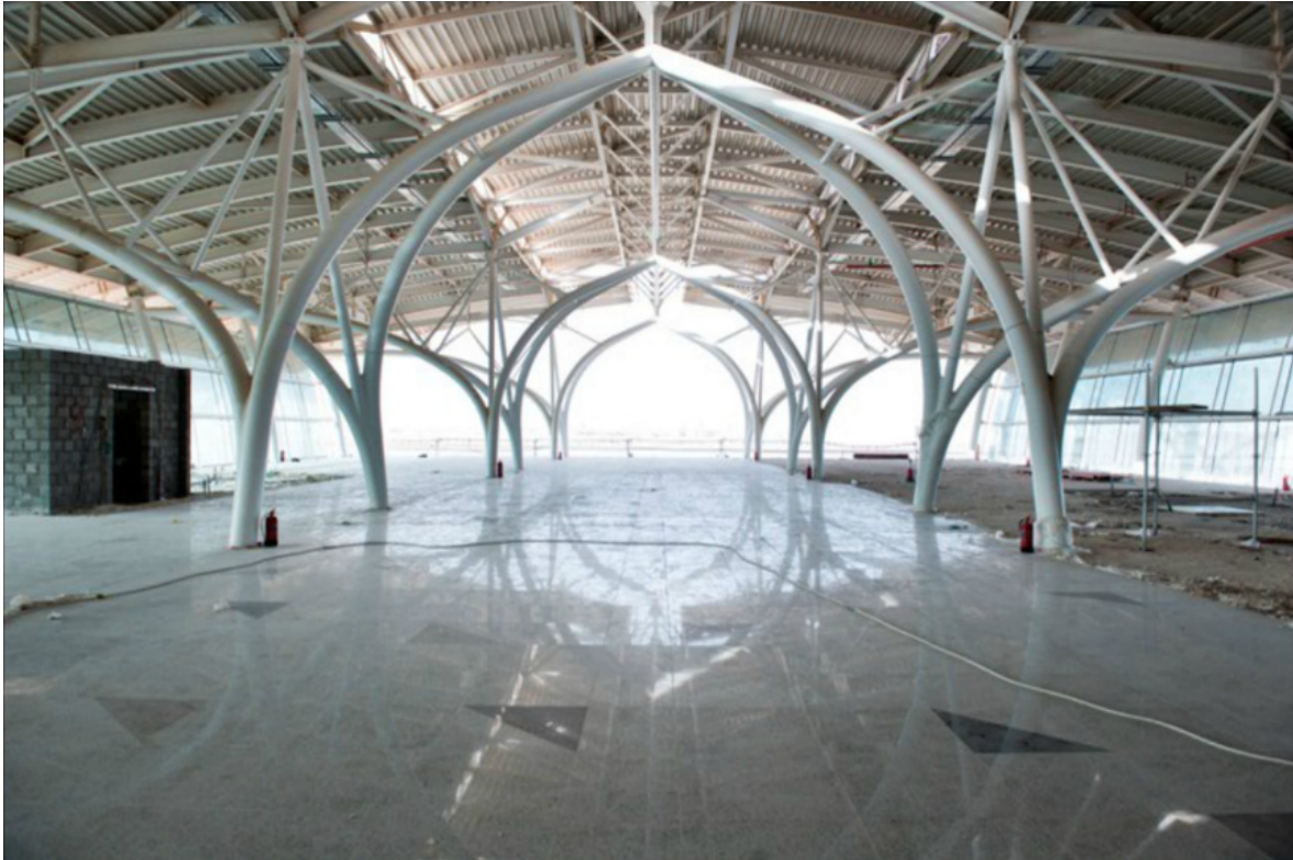
Figure 10. Cranes structures in position.
